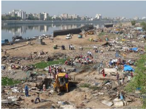
Image 8: Demolitions on the riverfront in November 2011 (photo by author)
