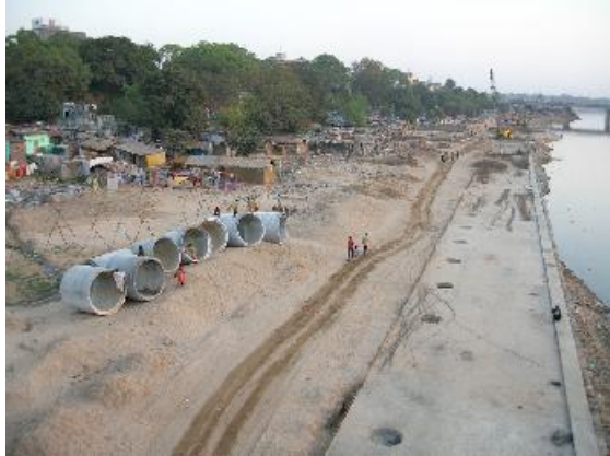
Image 4: Riverfront project construction / land reclamation in 2006 (photo by author)
